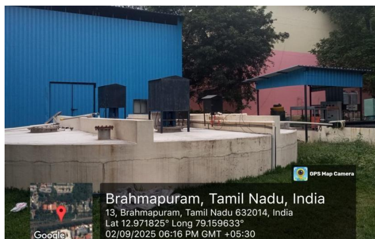
Figure 2.4 Photograph showing Bio-methanation Plant
