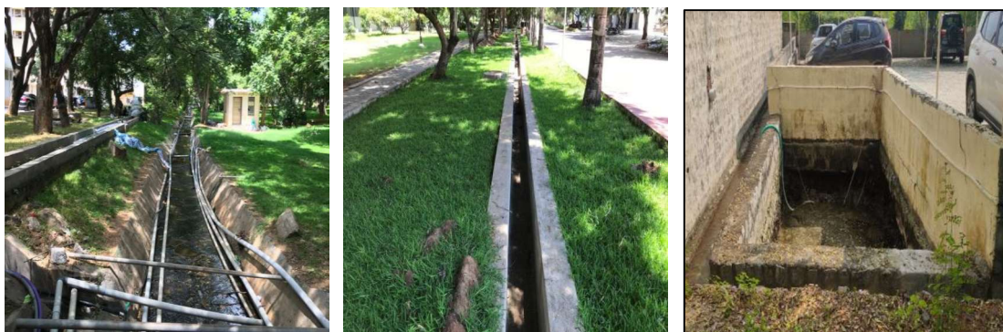
Figure 2.14: Photographs of Storm water drain
