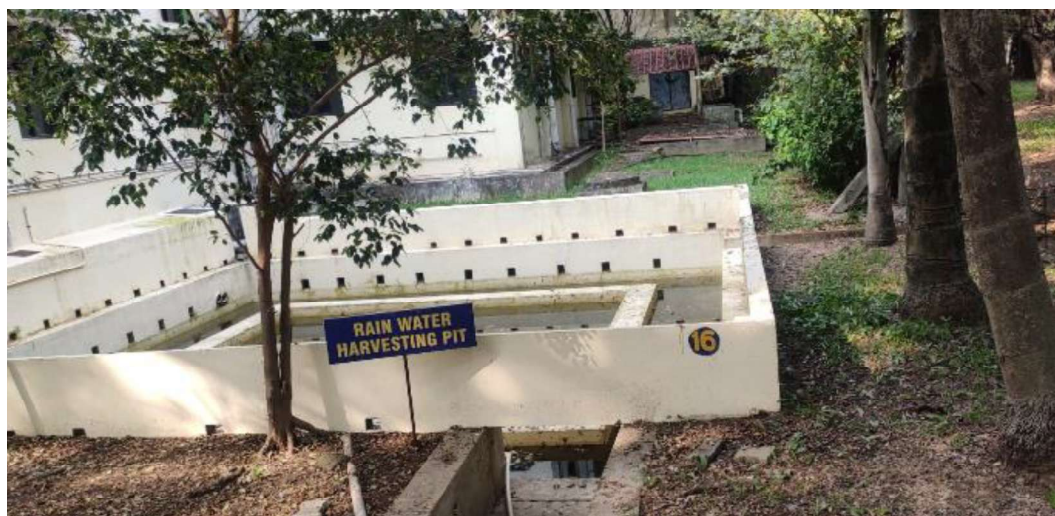
Figure 2.13: Photographs of Rainwater Harvesting Pit
