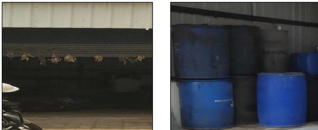
Figure 2.20: Photographs showing Used Oil is stored in MS Drums and HW storage Shed
