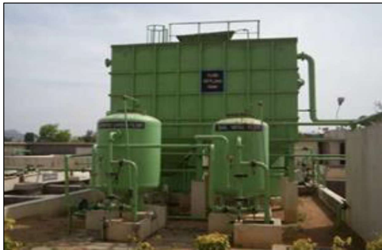
Figure 3.6 Photograph of bio mass plant
