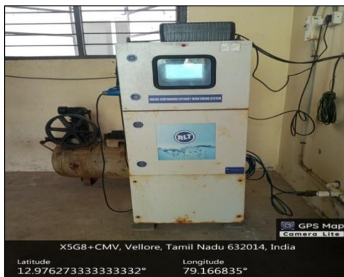
Figure 2.12: Photographs showing OCEMS installed at the outlet of STP
