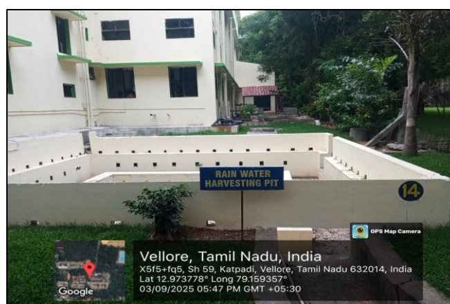
Figure 2.13: Photographs of Rainwater Harvesting Pit
