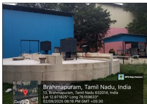
Figure 2.17: Photograph showing Biogas Plant
