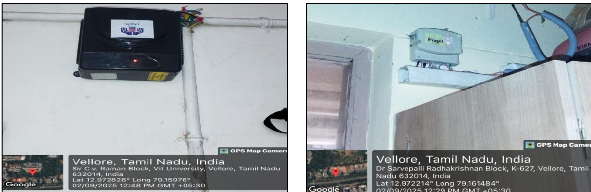
Figure 2.3 Photographs showing motion sensor based lighting system in Hostel blocks and Academic Buildings
