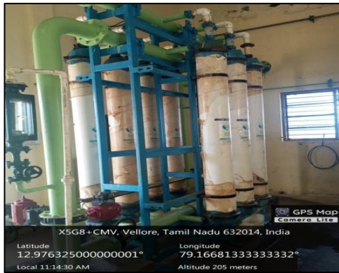
Figure 2.11: Photographs of Tertiary Treatment Units installed in STP
