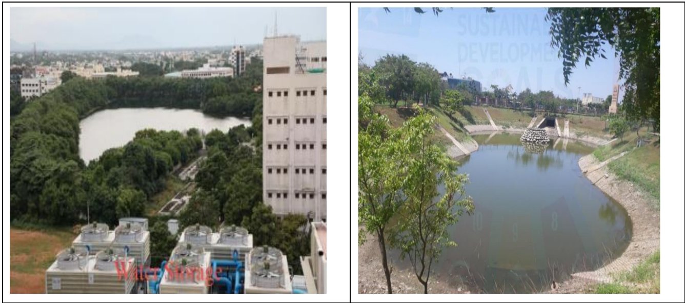
Photographs 20: View of Rainwater Harvesting Structures – VIT, Vellore
