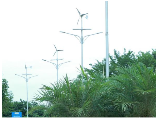
Fig.5 – Wind-powered exterior (pathway) lightings
