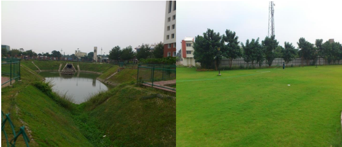
An artificial lake for Rainwater harvesting and Recycled Water used for Lawns
