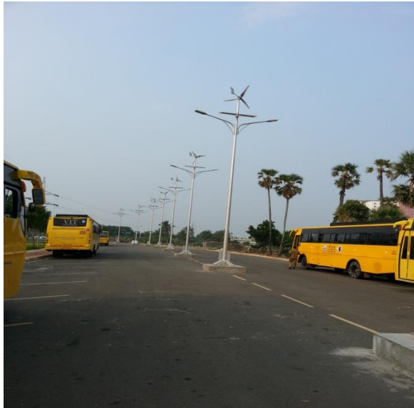
Hybrid type (solar & wind) street lighting
