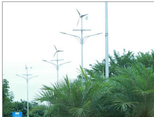
Wind-powered exterior (pathway) lightings
