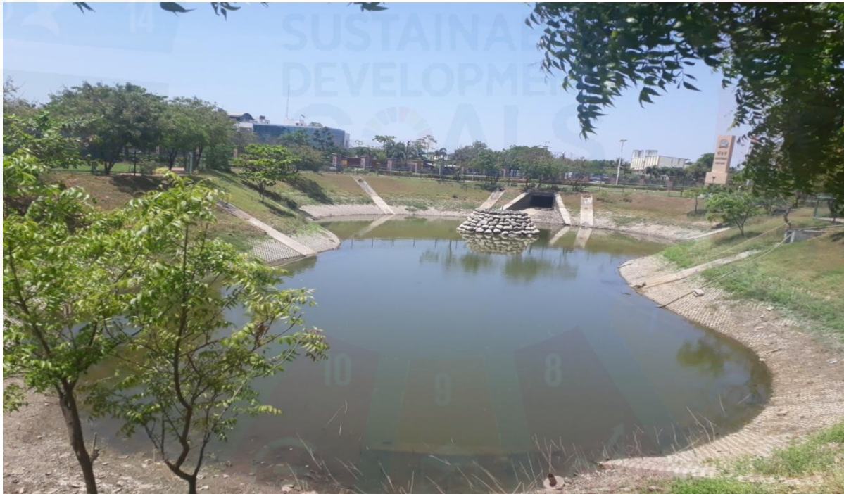
Rain Water harvesting pond
