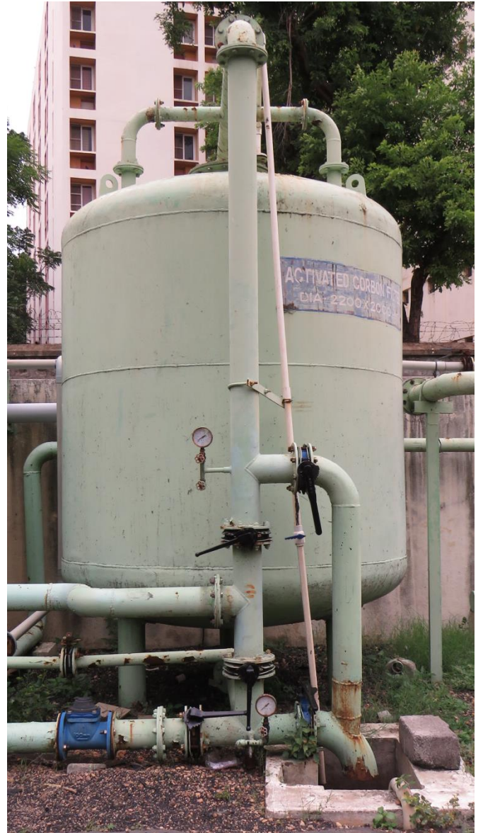
Sewage Treatment Plant Output Meters
