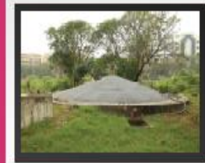
BIO GAS PLANT
