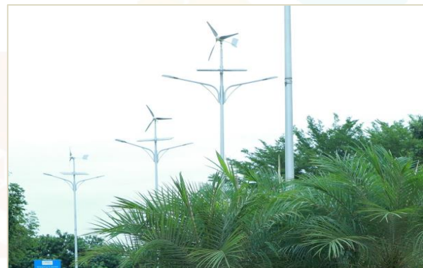
Solar and wind powered LED street lights
