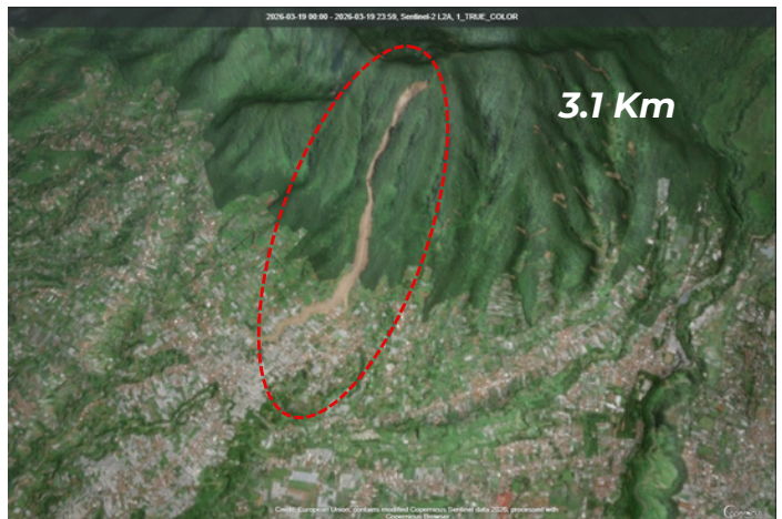
After Landslide (19 Mar 2026)
